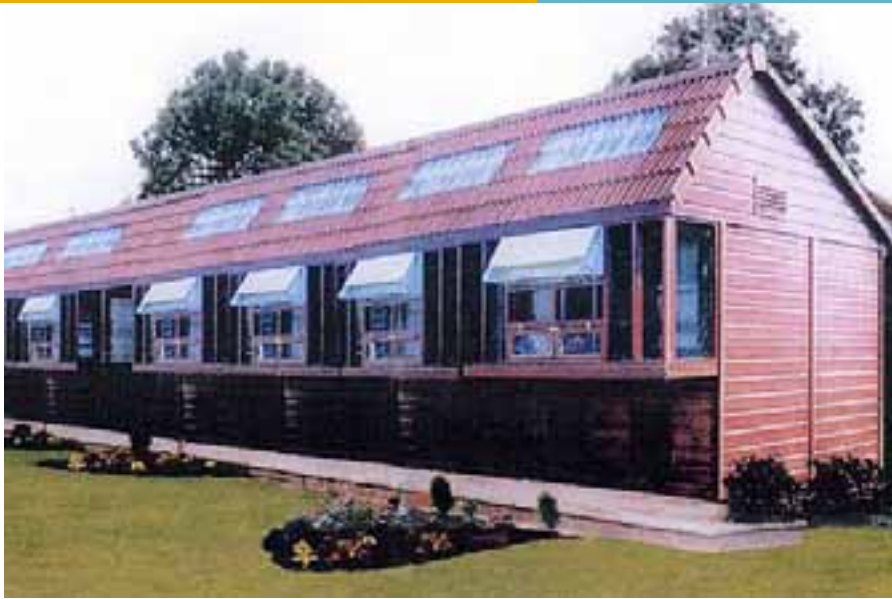
The new loft is designed to maximise the amount of natural light so the birds can sunbathe
